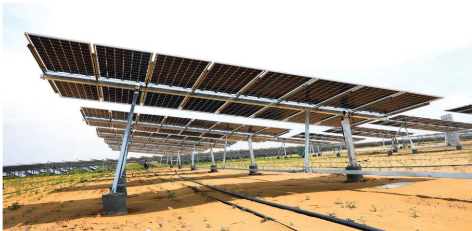
Figure 6 Sketch Map of Installation of Bifacial Module
